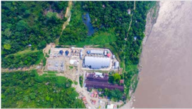
The Iquitos power plant
